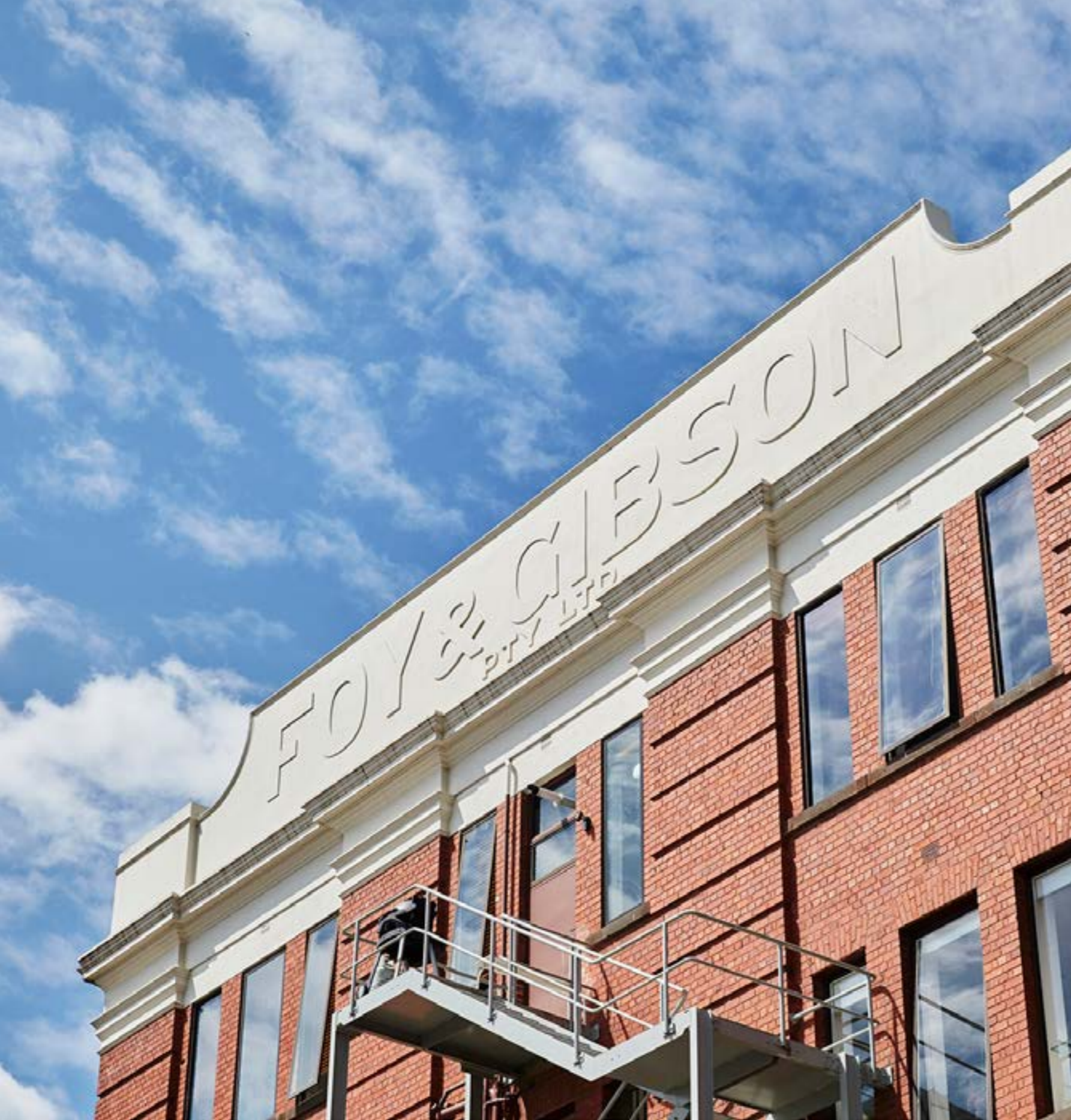
05 Foy & Gibson, 76 Oxford Street, Collingwood Property X Building Management.
